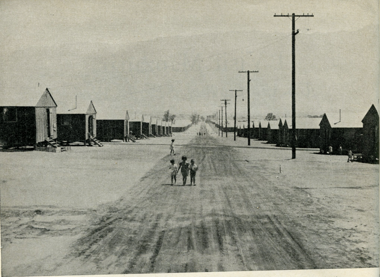
MANZANAR RELOCATION CENTER, MANZANAR, CALIFORNIA. Street scene of barrack homes at this War Relocation Authority center. The windstorm has subsided and the dust has settled.
